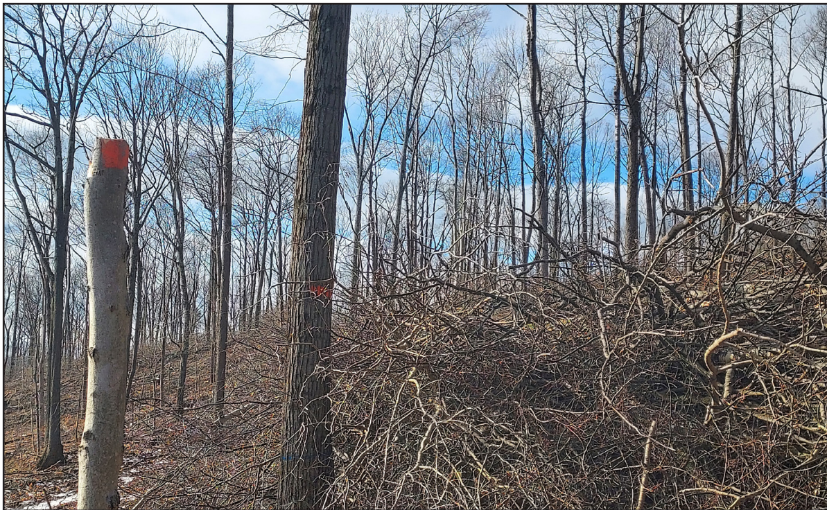
Figure 9: Following on the example given by Kellen Murphy, at the Arnot Forest we used a paint roller and telescoping handle to position marks indicating wall height. In this example, the logger removed the upper portion of the beech trees for use in building the slash wall.
