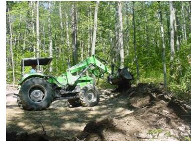
At times it may be possible to install a pool or pond as part of an ongoing timber harvest or other activity. Skid trails that will be abandoned can provide the opportunity to create a woodland pool. By dropping the blade on the bulldozer, a logger can excavate a shallow 1-2 ft depression that can develop into a shallow pool.
