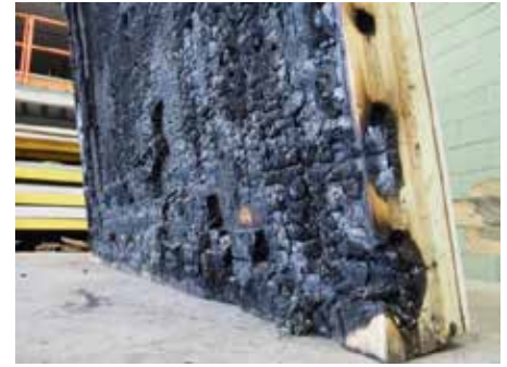
Wall assembly after testing showing the depth of charring on the exposed side. NRC (2014) Fire Endurance of Cross-Laminated Timber Floor and Wall Assemblies for Tall Wood Buildings.
