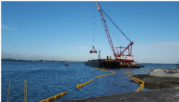
Figure 1. As a post-review discovery, underwater excavation from two boats was simultaneous with large-scale dredging, as seen here looking south in San Juan Harbor. In zero underwater visibility, the boom of the dredge hitting the seabed was unforgettable. Additionally, we had to work around frequent barge arrivals and departures.
