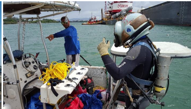
Figure 2. Hard-hat diver getting ready to fill the lift bags for raising the shipwreck to mid-water, for relocation.
