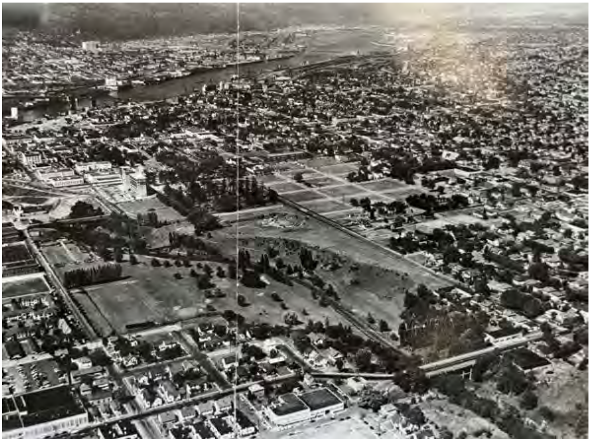
Looking NW, 1952. The Department of Interior Building (now Bonneville Power Administration), is under construction. It is the first large building under construction in the Lloyd District.
