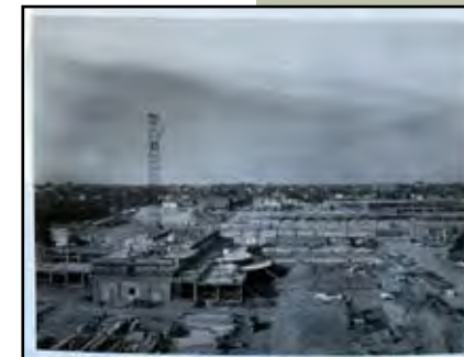
Construction of mall and hotel underway
