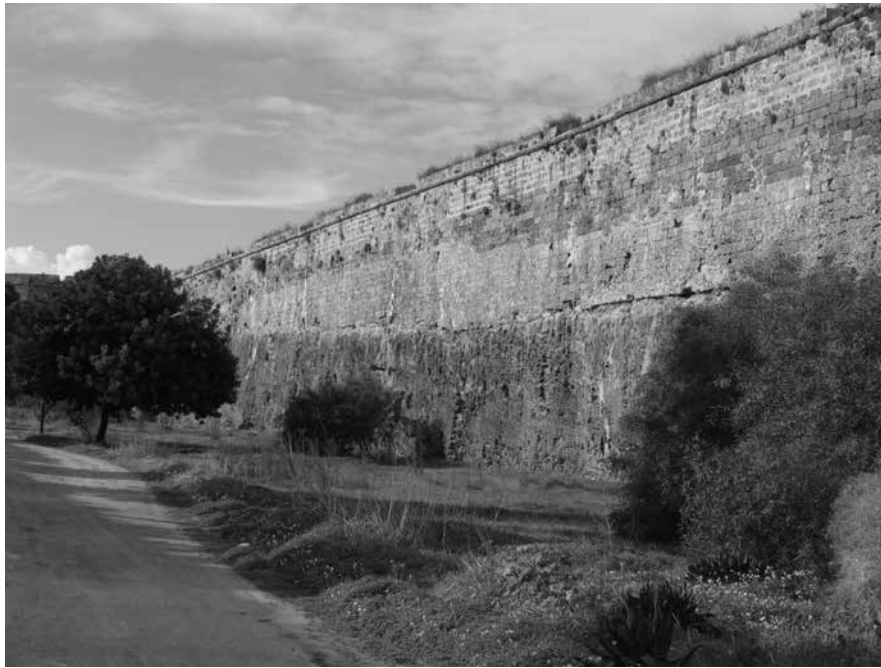
FIG. 3. Section of the walls of Famagusta between the ravelin and the Santa Napa Bastion with natural excavated rock making up the lower sections (photo by author).
