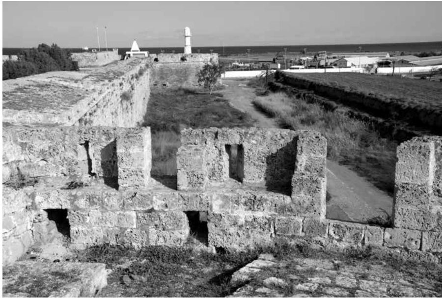
FIG. 5. Andruzzi Bastion crenellations, looking east, with adaptations to the crenellations for firearms and artillery (photo by Dan Frodsham).
