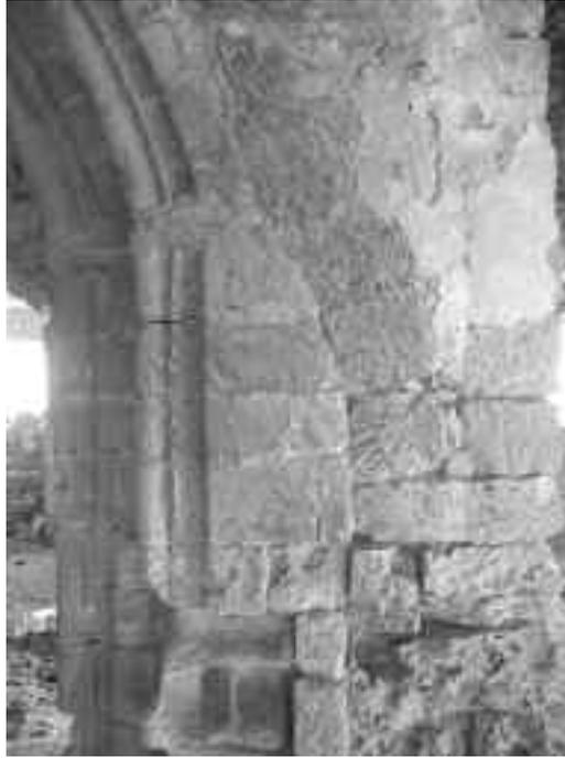
*Fig. 5: Piers of the 14<sup>th</sup> century dome, showing seam between the original masonry and masonry added in the 16<sup>th</sup> century*
