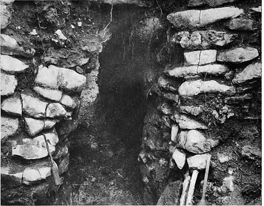
FIGURE 12. Sandstone arch in front of the niche. Gros-Guignon furnace. The keystone can just be seen at the top, and the base stones at the bottom. Observe the sandstone paving.
