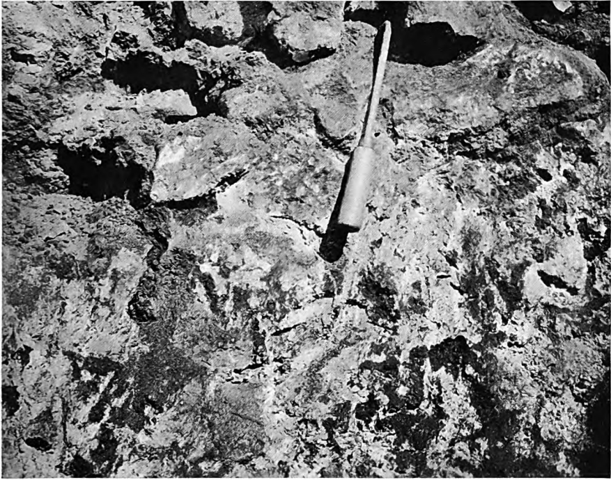
FIGURE 11. Lower masonry of Gros-Guignon furnace. Above, blocks of flint packed with red earth; below, sandstone masonry with the external face calcined to plaster.
