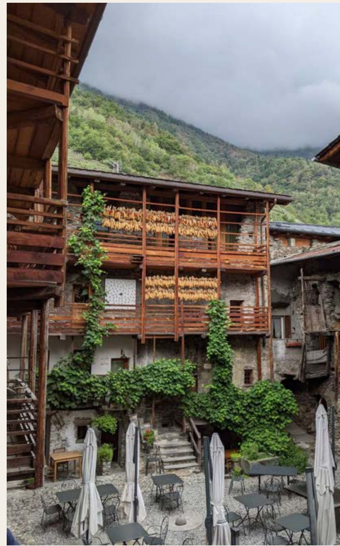
Restored buildings in Teglio
