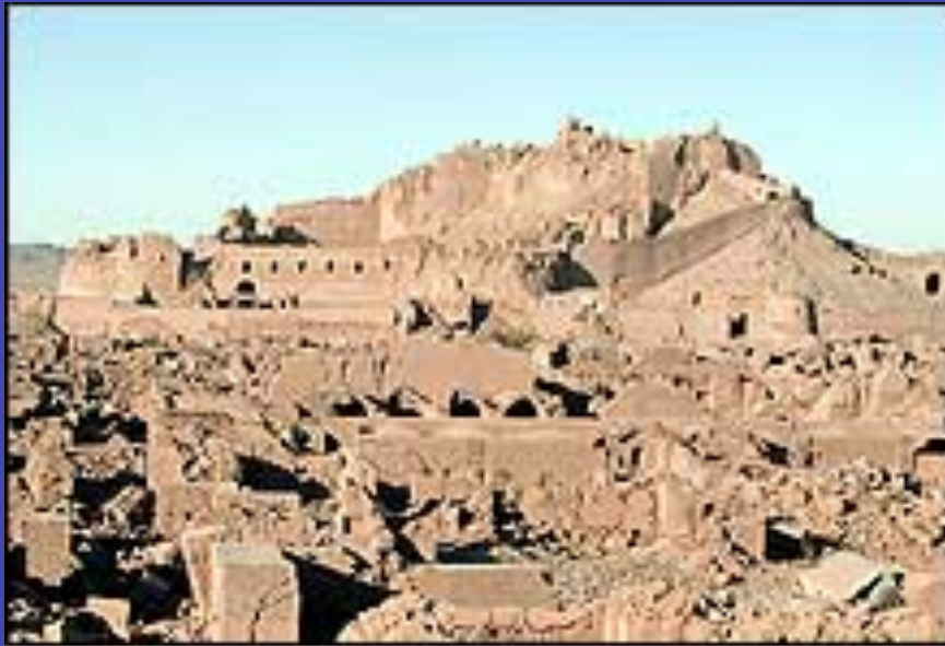
Collapsed adobe buildings
