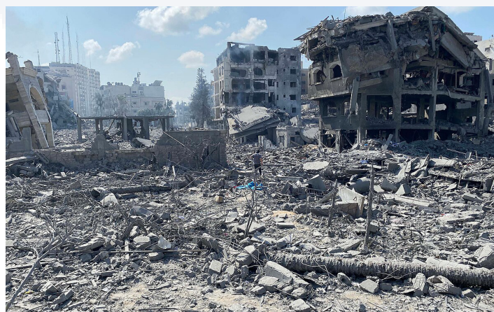
Israeli airstrike destroys buildings in Gaza City on October 9, 2023. (Photo courtesy: Wikimedia Commons)
