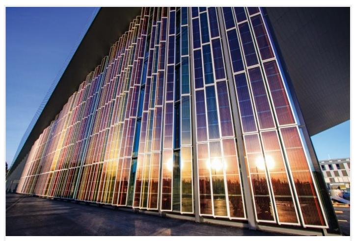
The colors of the SwissTech Convention Center come from dye-sensitized solar cells integrated into the facade in panels made by Solaronix.
