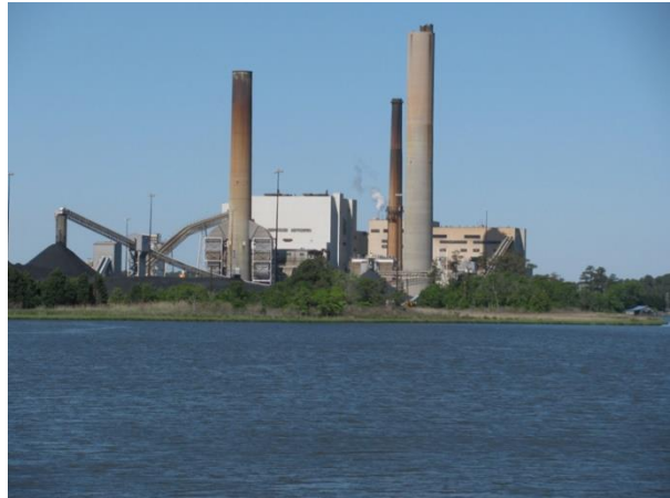
Figure 3: Power Plant Built Near Water Source
