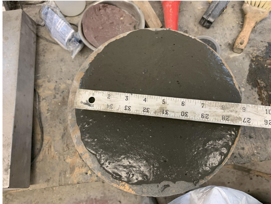
Figure 25. Measuring UHPC spread during a flow test.
