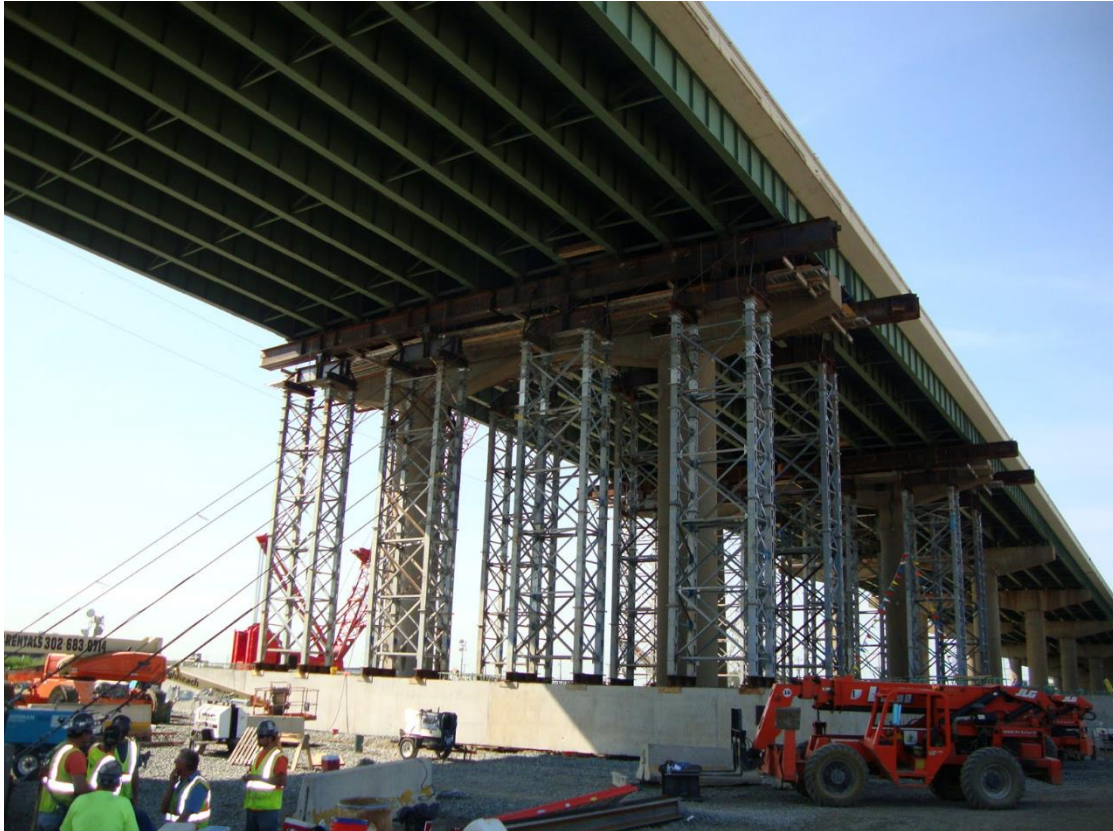
Figure 3-6 Proposed Foundation Repair & Temporary Support Elevation (Benton, 2014)
