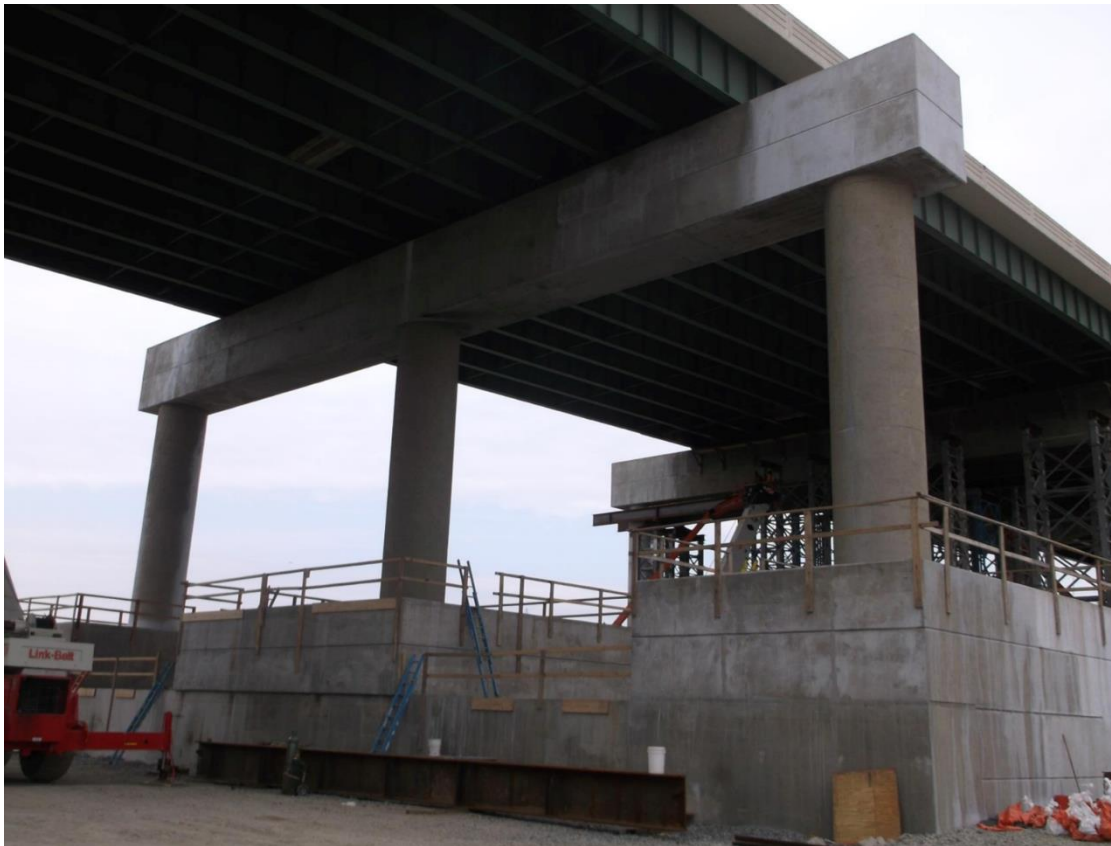
Figure 3-9 Permanent Completed Repairs (Benton, 2014)
