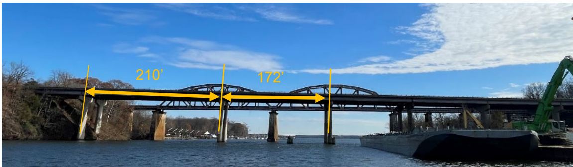
Figure 26. The bridge and the monitored spans with their length from the harbor deck's view
