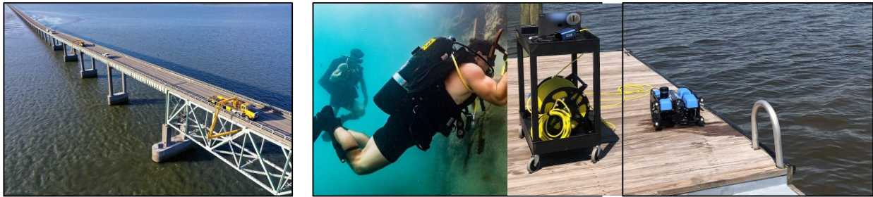
Figure 1. Hydraulic bridge and snoop truck [2], inspection dive team [3], and inspection ROV.
