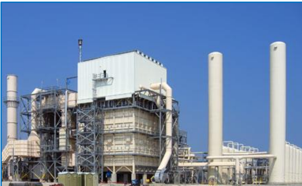
Figure 1: Steam Methane Reforming Plant - Linde Engineering
