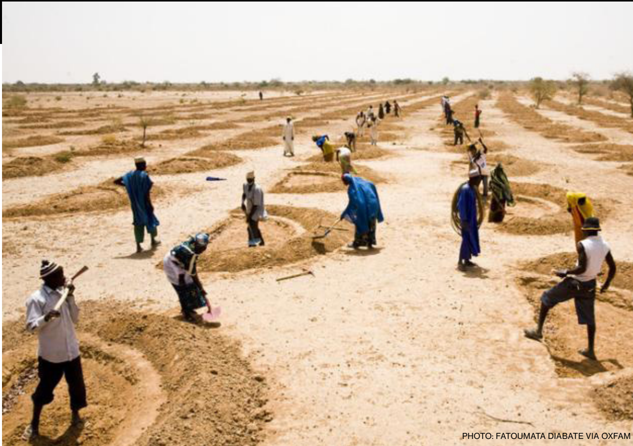
Construction of demi-lunes, a rainwater harvesting technique in the Sahel.
