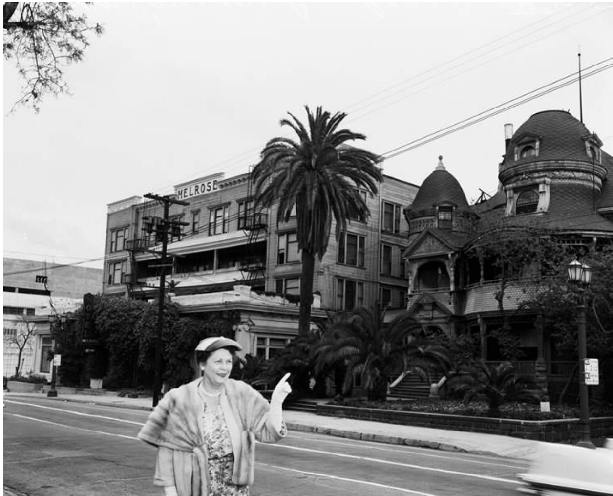
Figure 1.4. Existing conditions on Bunker Hill, 1957. In the foreground is Mary Connor Rasche, whose father designed the Melrose Hotel, pictured at rear. Source: USC Libraries, Los Angeles Examiner Collection, File Name: EXM-N-12099-002~2.tiff.
