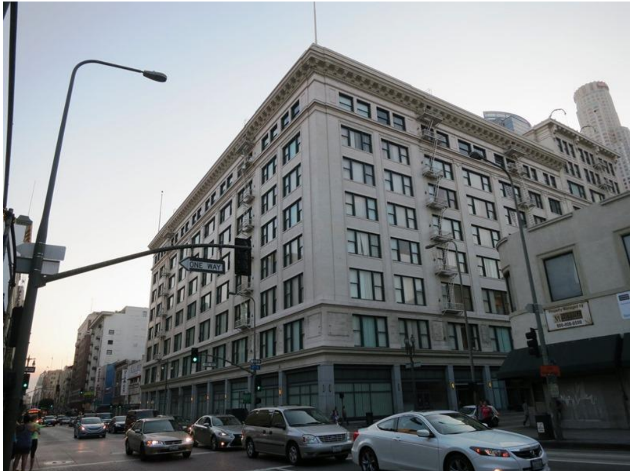
Figure 3.8. Present-day view of the Junipero Serra State Office Building, view looking southwest. Photo by author.
