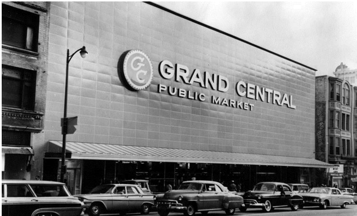
Figure 2.5. Tiled veneer obscures the historic façade of the Lyon Building, 1962. Source: Los Angeles Public Library, Order Number 00033764. Permission requested – request pending.
