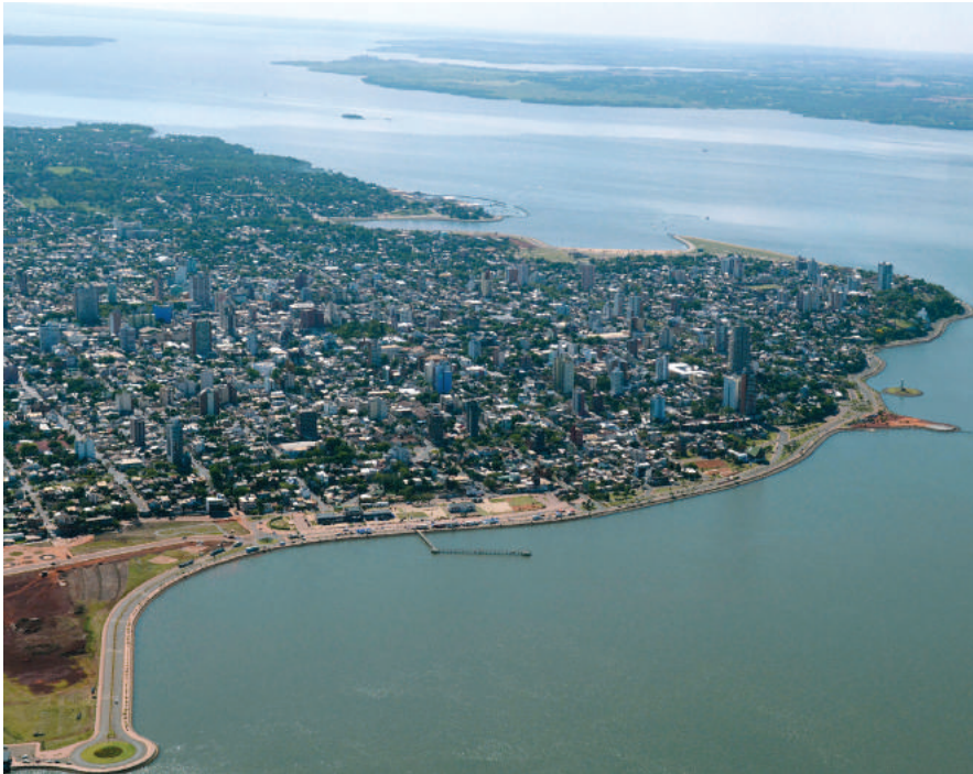
An aerial view of the hydroelectric plant; the Guarani worry about bad waters.
