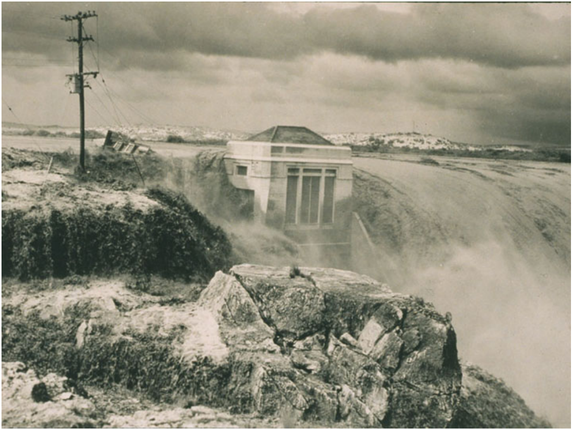
Figure 16. On June 24, 1948, the Devils River is seen pouring over Lake Walk Dam near Del Rio, Texas (Photo from Breeding 1948, USGS 61). Peak discharge was measured at over 441,000 cfs after nearly 21" of rainfall fell in this region in a 48 hour period.
