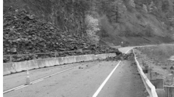
Rockfall, Estacada fire: Oregon Department of Transportation
