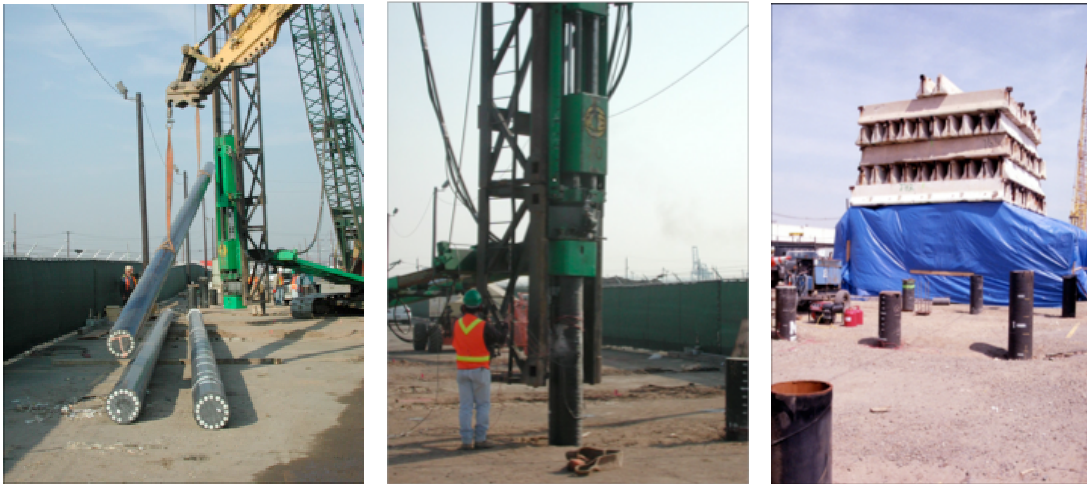
Fig. 1. Photographs of Installation and Load Testing at
