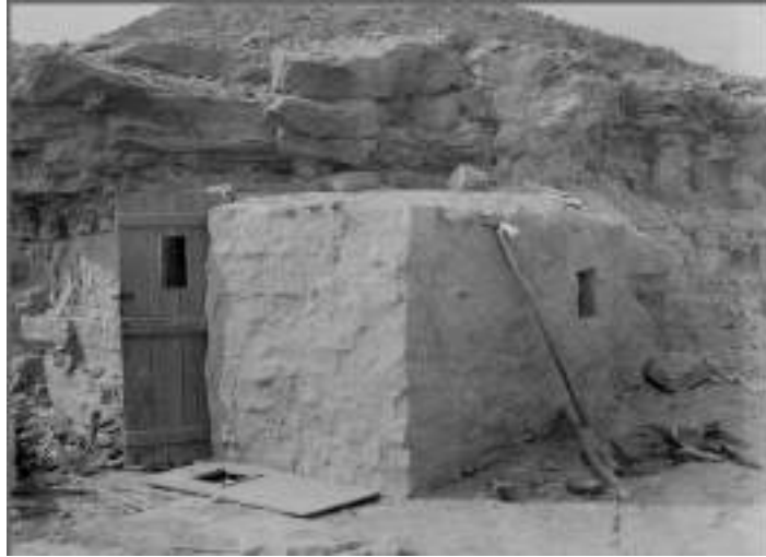
Fascist Blockhouse on Purberell Hill, ALBA PHOTO 11-1121, Tamiment Library, NYU
