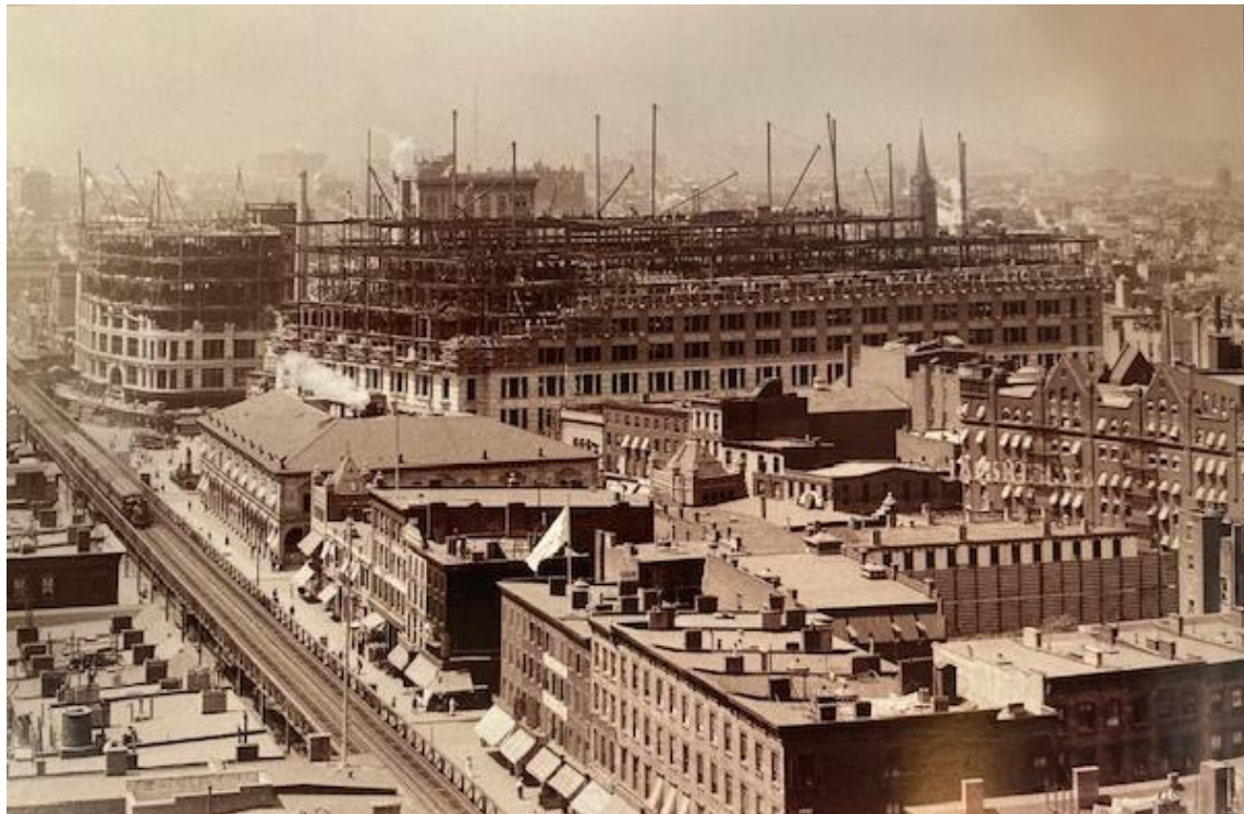
1 Construction of "east" building in 1902
