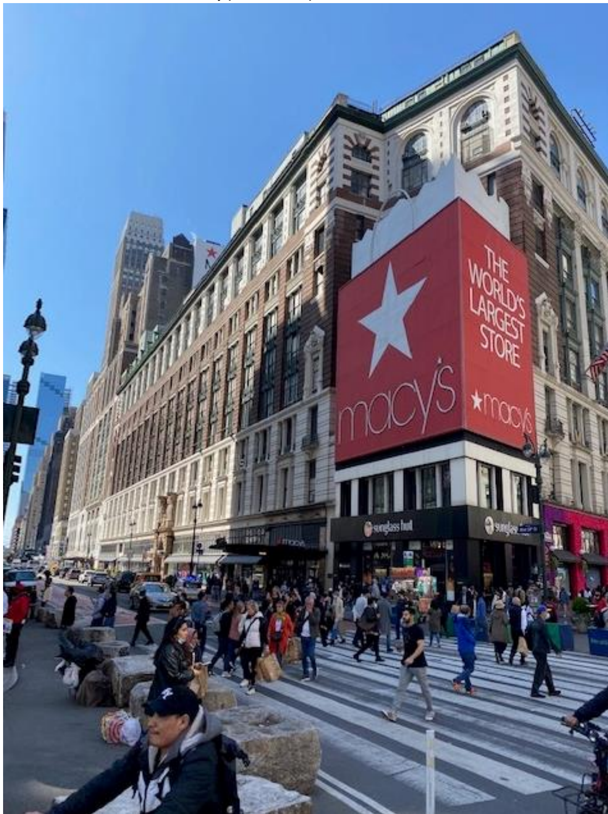
Corner of 34 th street and Broadway (The “Notch”)
