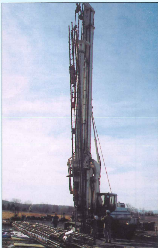
Rig leads cage for placement.
