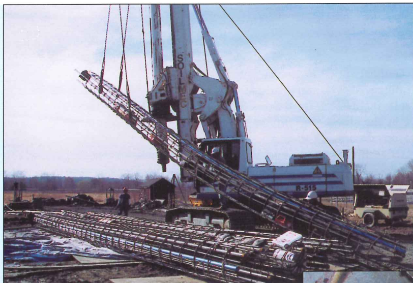
Cage to be placed in Test Shaft.
