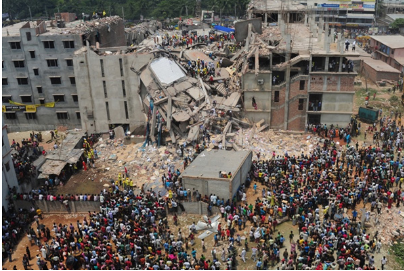
Image 3. The collapse of the Rana Plaza building that housed garment factories, killing 1,134. Munir Uz Zaman/Agence France-Presse — Getty Images, 2013.
