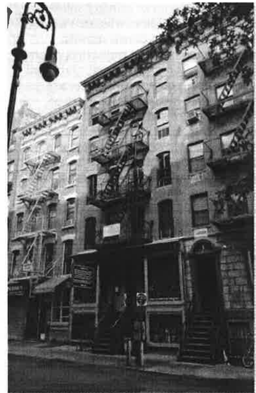
Fig. 1. Façade of 97 Orchard Street. Shop Life is located in the basement level of the building. Photo by Keiko Niwa
