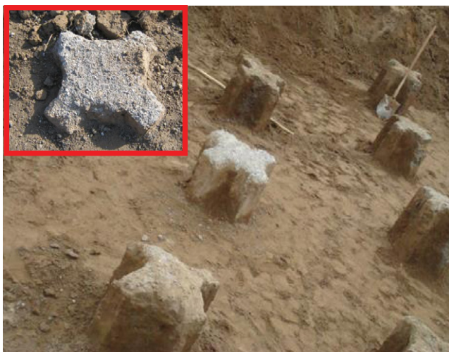
Figure 2. Typical XCC pile in the field
