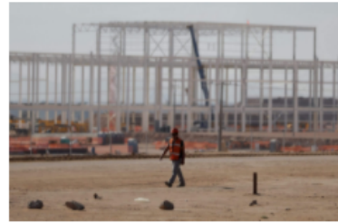
A construction site for a planned factory outside of the US.
