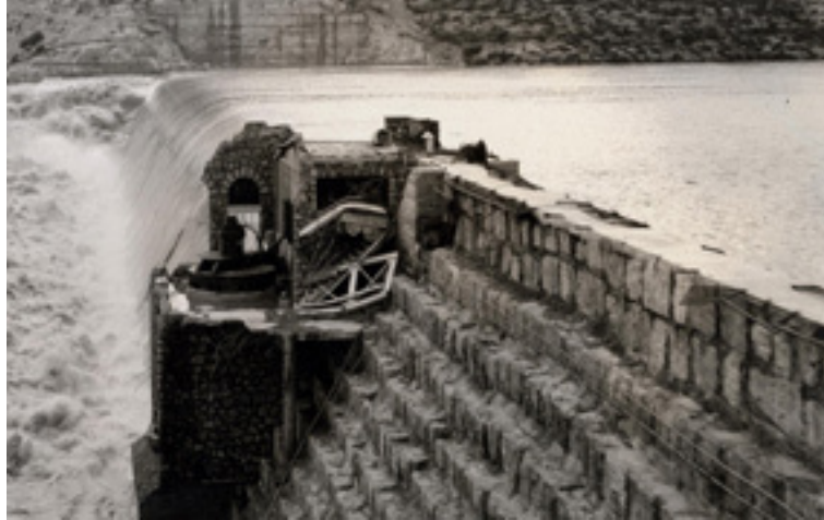
Figure 11711 Devils Lake Dam (National Park Service [NPS], n.d.)
