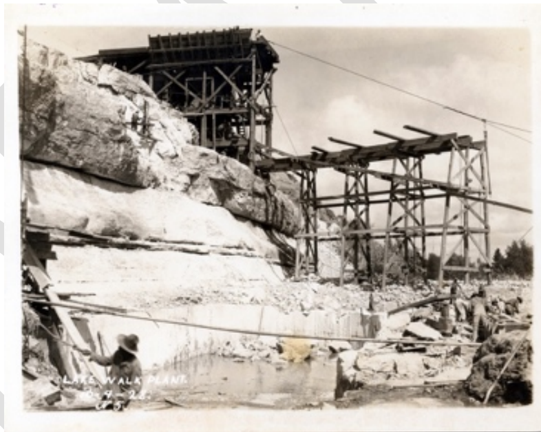
Figure 12812 Lake Walk Plant Construction (NPS, n.d.)
