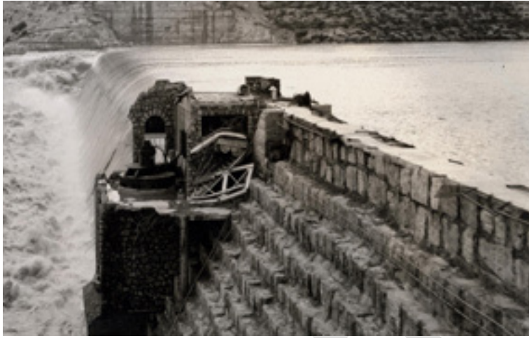
Figure 11. Devils Lake Dam (National Park Service [NPS], n.d.)
