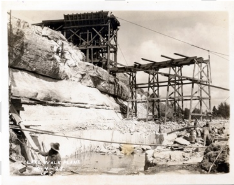
Figure 12. Lake Walk Plant Construction (NPS, n.d.)
