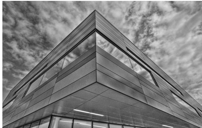
In January 2010 work began on the Campus Recreation Center. It opened in October 2012 and provides meeting space for sports clubs, more than 50 classes a month, and top-of-the-line exercise equipment.
